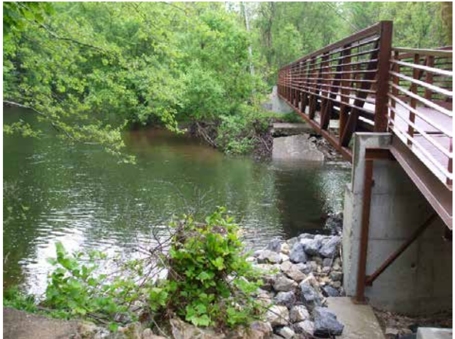
Pedestrian bridge and trail over Rapps Dam.
