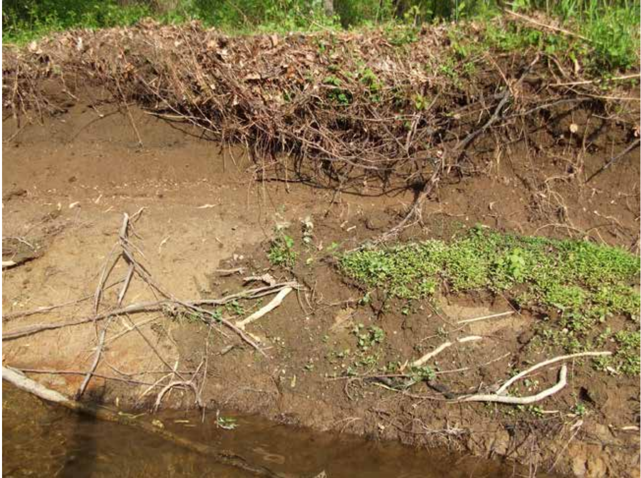
Eroding bank at Site 18 on mainstem showing grayish layer and charcoal
