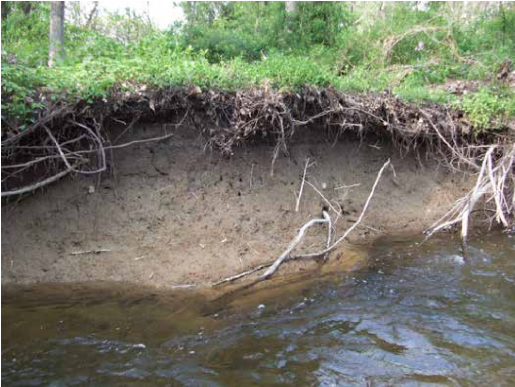
Eroding banks at site 18 on South Branch
