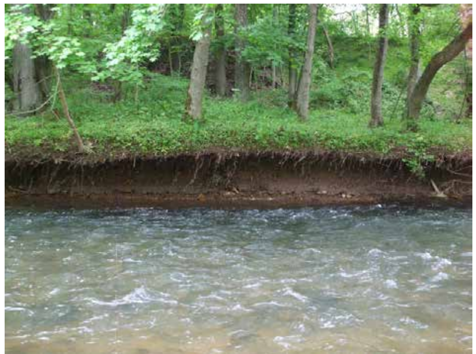
Terrace above Rapps Dam showing horizontal layers and stranded vegetation.
